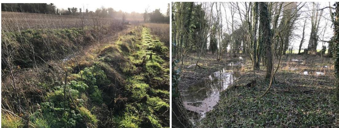
Plate 5 Embanked nature of Dane Hill Watercourse towards the A11 (left) and wet woodland further upstream (right)
