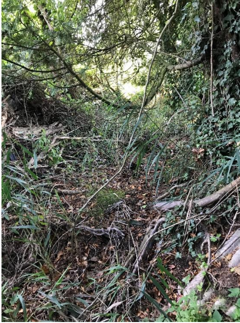
Plate 13 Nature of watercourse at the location of Option 1 for the Burwell National Grid Substation Extension
